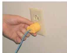
Extension Wire with Cable Connected Only to Ground Contact
