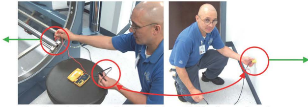
Measuring Resistance Between Chamber and Building Common Ground
